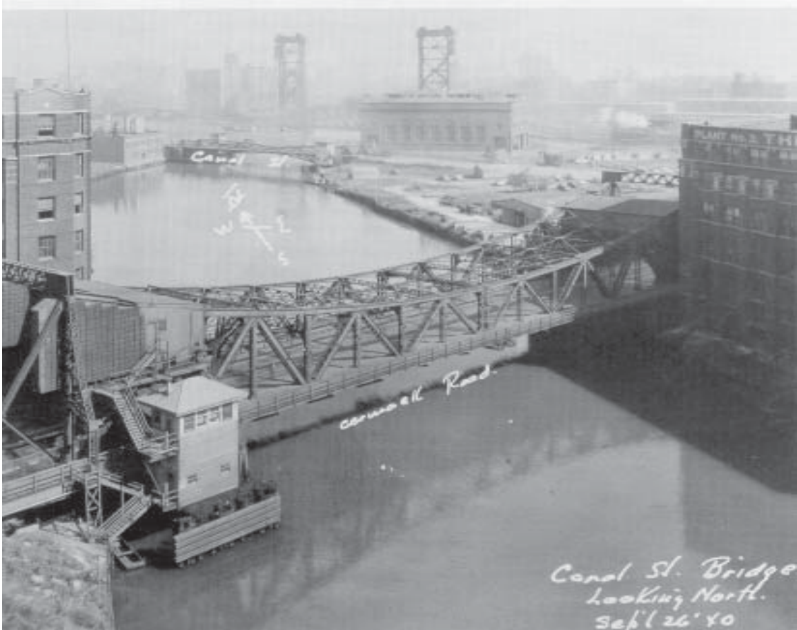
Below: A historic view of the district looking northeast. The Thomson & Taylor Building (left), the Cermak Road Bridge, and the Hoyt Building (right) are seen in this photo from 1940. Pennsylvania Railroad Bridge 458, a vertical lift bridge constructed in 1915, is seen in the distance. The bridge is located just south of 18th Street and east of Canal Street.
