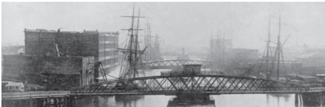
Bottom: The Lake and Randolph Street bridges are seen here in the mid-1860s. Land travel was often delayed by the cumbersome swing bridges which pivoted on a center pier to provide a narrow passage for ships.
